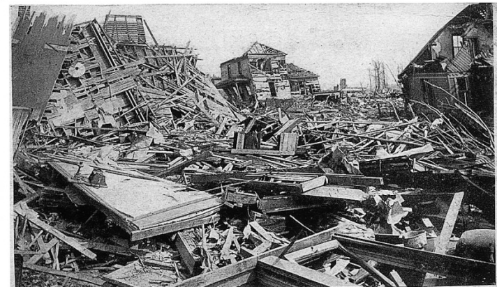
HOMES SHATTERED TO PIECES AT MURPHYSBORO, ILL., IN TORNADO OF MAR. 18, 1925, WHICH RENDERED HOMELESS HALF THE POPULATION OF THE CITY. ABOUT 1200 HOMES WERE COMPLETELY DESTROYED IN AN AREA 1 MILE WIDE AND 2½ MILES LONG.
