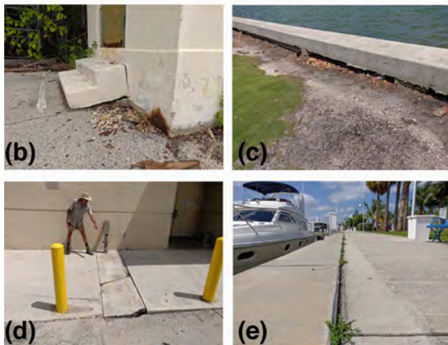
Figure 2. (a) Location map of our study area in southeast Florida based on a ©Google Map imagery. The map shows the location of documented coastal subsiding areas and planned GPS sites. Insert shows the location of the study area with respect to state of Florida. (b) Subsidence-induced structural damage to a building in Matheson Hammock Park. (c) Observed subsidence along seawall in Morningside Park. (d) Subsidence-induced structural damage at the entrance to the Kovens Conference Center at the Biscayne Bay Campus of Florida International University (FIU). (e) Observed subsidence along seawall in Haulover Park.
