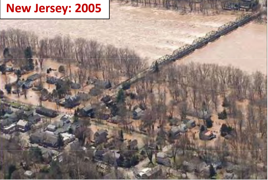
Flooding in the Study Area, April 2005
