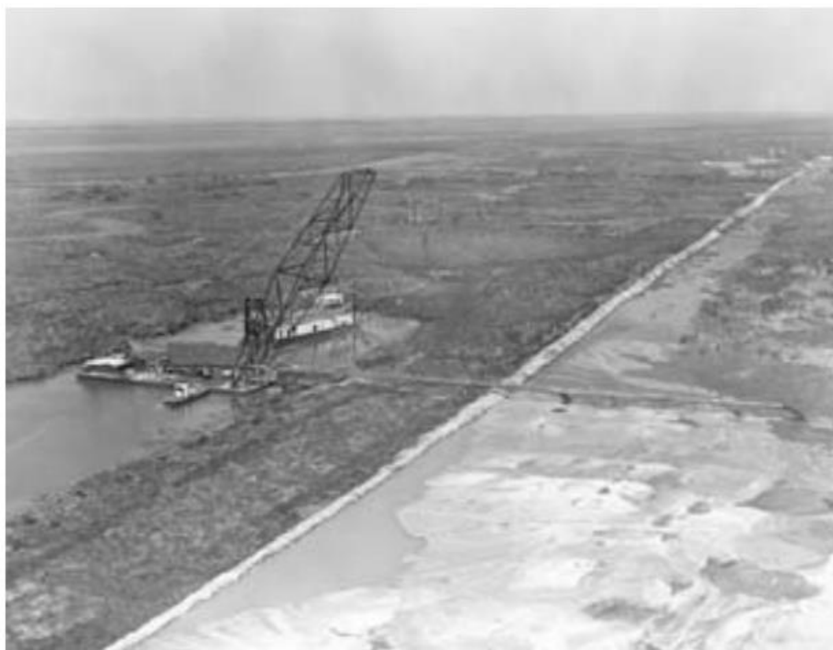
The Kissimmee River was “channelized” to manage its water flow. Over the course of nine years (1962-1971), the meandering river was cut and dredged into a straight canal (C-38) with six water control structures. Two-thirds of the original floodplain was drained ( https://www.sfwmd.gov/sites/default/files/documents/bts_krr_phase_1.pdf )
