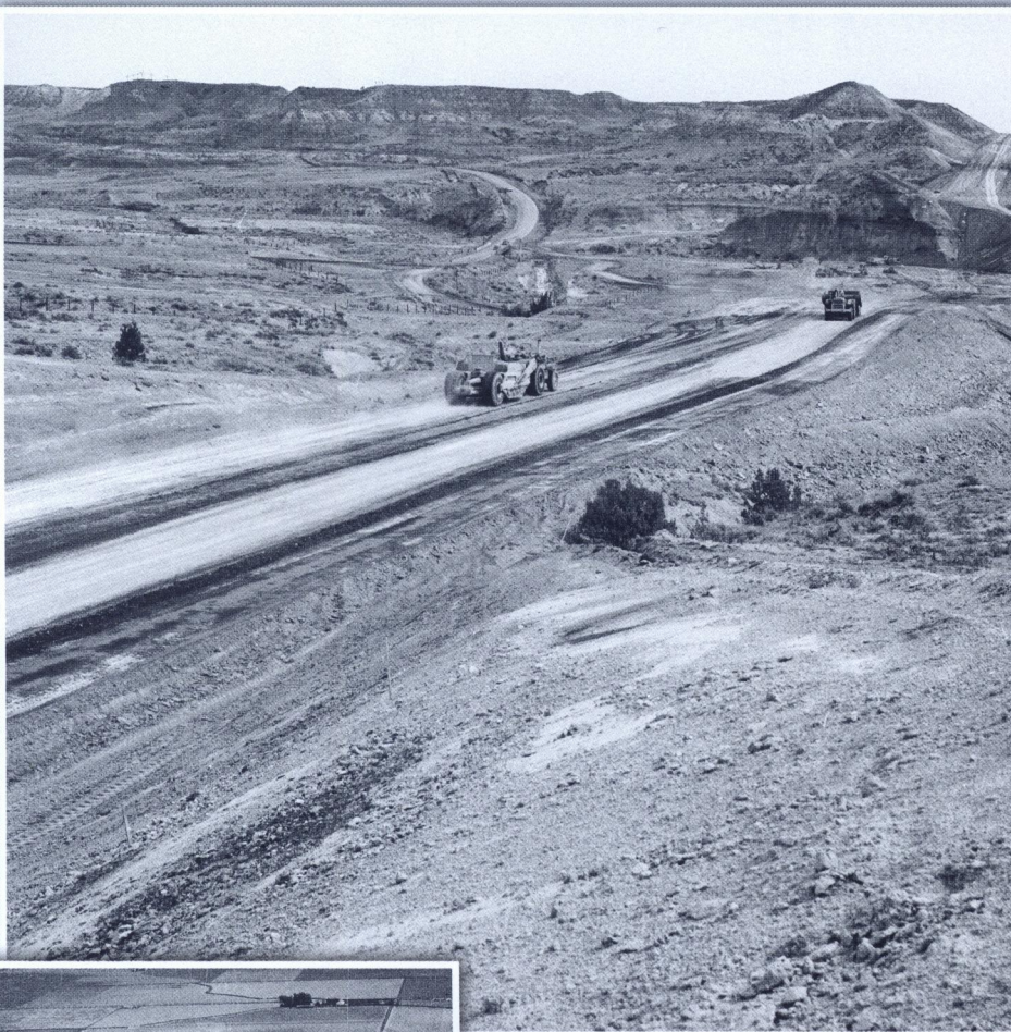
← Scrapers move earth on an I-94 construction site west of Miles City, August 22, 1960.
