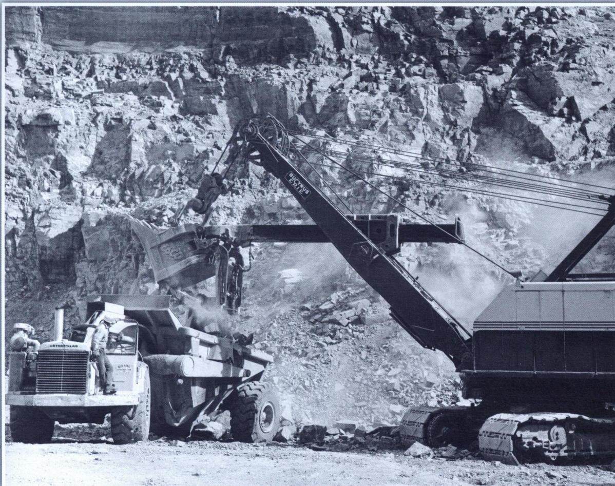
↑ A cable shovel fills a haul truck with debris from blasting, March 23, 1962.
