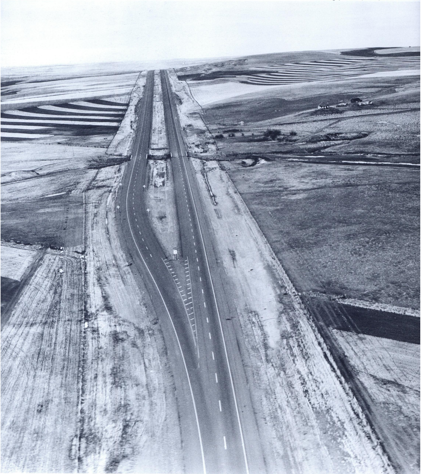
The original interstate plan envisioned a nationwide two-lane system, switching to four lanes only in the vicinity of cities. In Montana, however, planners surmised that the federal government would eventually require four-lane interstates and acquired three-hundred-foot corridors in anticipation of the expansion. Above, two lanes split into four on I-15 near Ulm as the highway approaches Great Falls in 1959.
