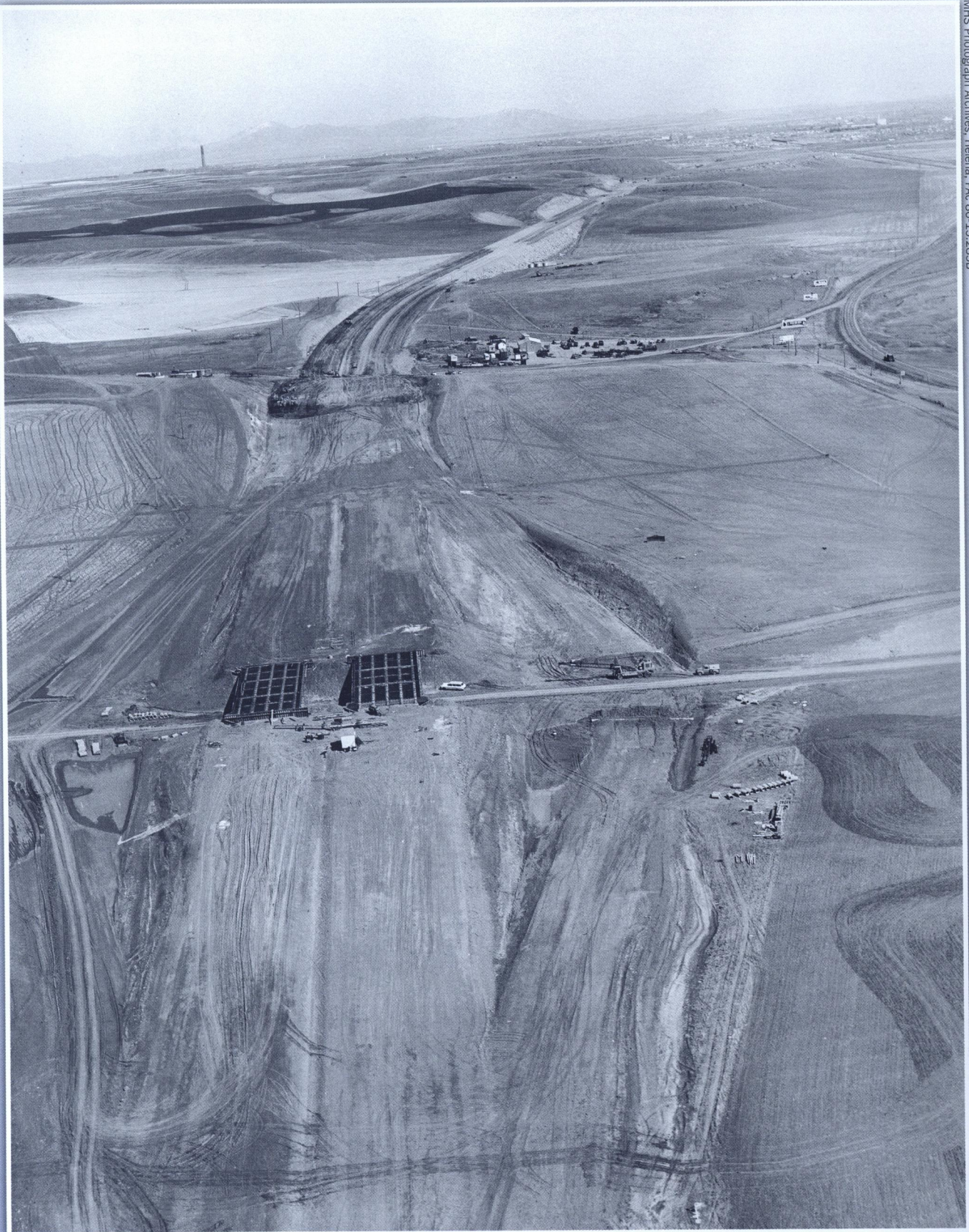
↑ The layout takes shape for the Manchester I-15 interchange between Great Falls and Vaughn. The gridlike platforms in the center are the substructure and beams for the overpass. In the distance, Great Falls, the Highwood Mountains, and the Anaconda Company smelter stack are visible.
