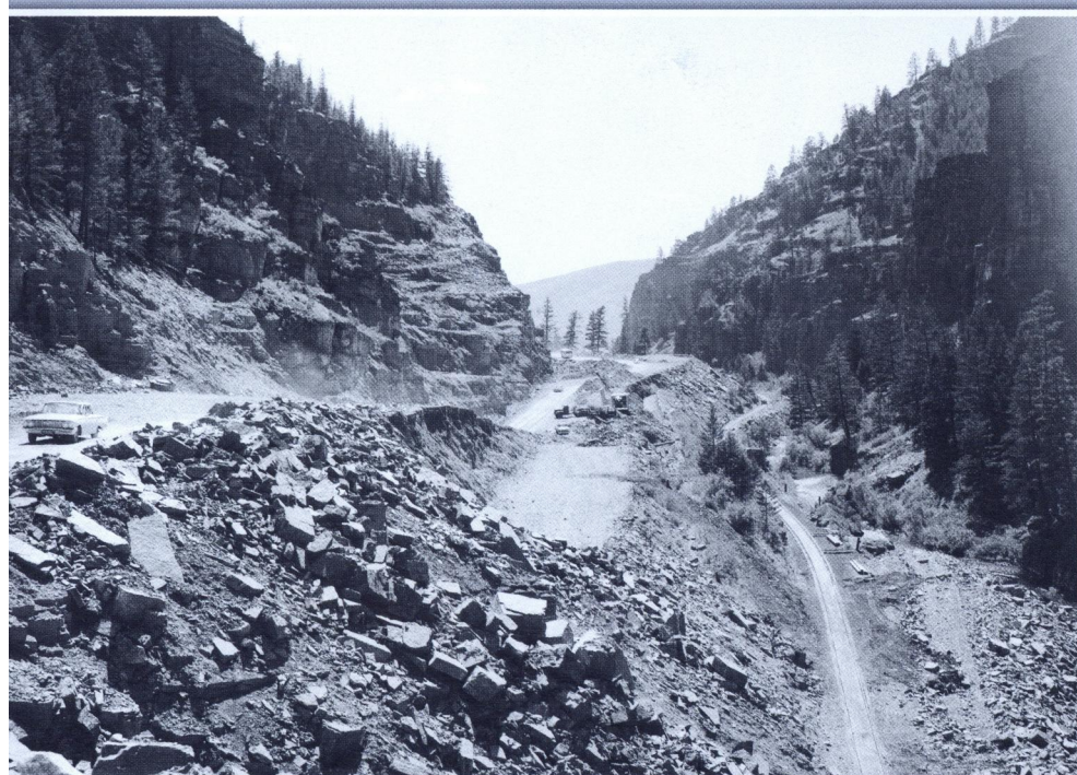
← The southernmost 3.4 miles of the interstate through the Wolf Creek Canyon was the first Montana section to cost more than $1 million per mile. Here, the new highway route is shown above the railroad bed and Little Prickly Pear Creek in summer 1962.
