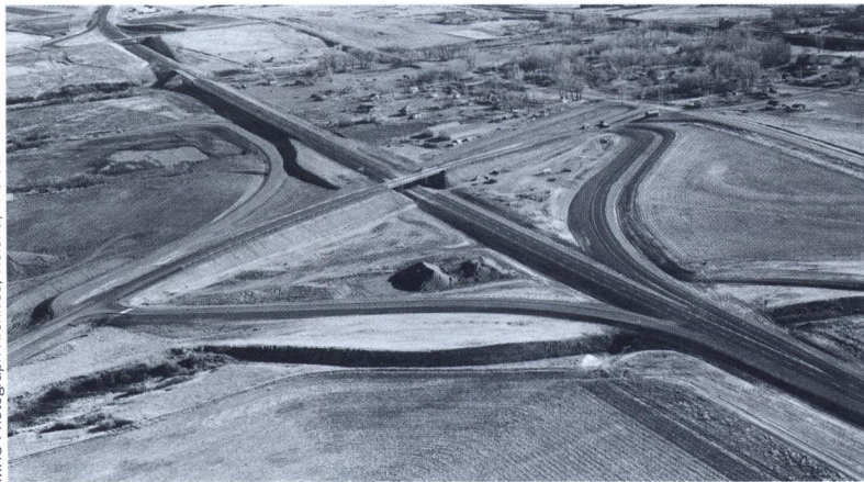
By the mid-1960s, all interchanges, whether cloverleaf or diamond pattern, had to meet strict geometric standards, and all overpasses had to accommodate a fourteen-foot overhead clearance. Pictured here on November 30, 1962, the west Wibaux interchange on I-94 shows the half-diamond variation used only four times on Montana interstates. With two half-diamond interchanges, one on each end of town, drivers had to exit at one end and reenter the interstate at the other.
